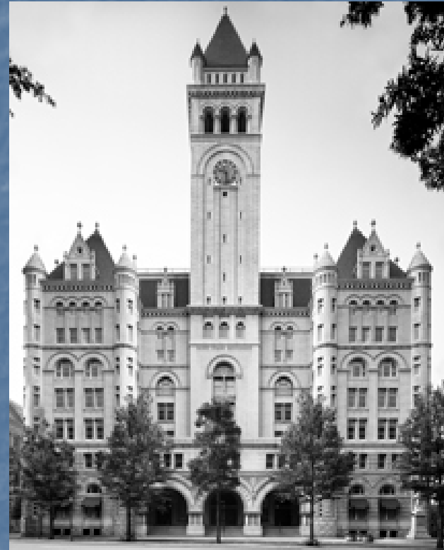
Old Post Office Pavilion 1100 Pennsylvania Avenue NW Washington, DC 20506
