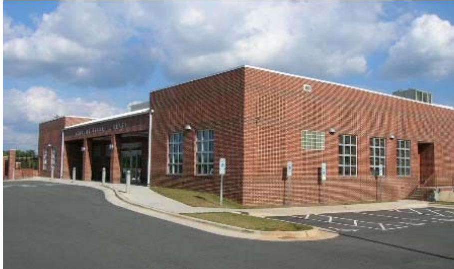
Fig. 1. Hemphill Branch Library-Exterior. Image courtesy of Hemphill Branch Library.
